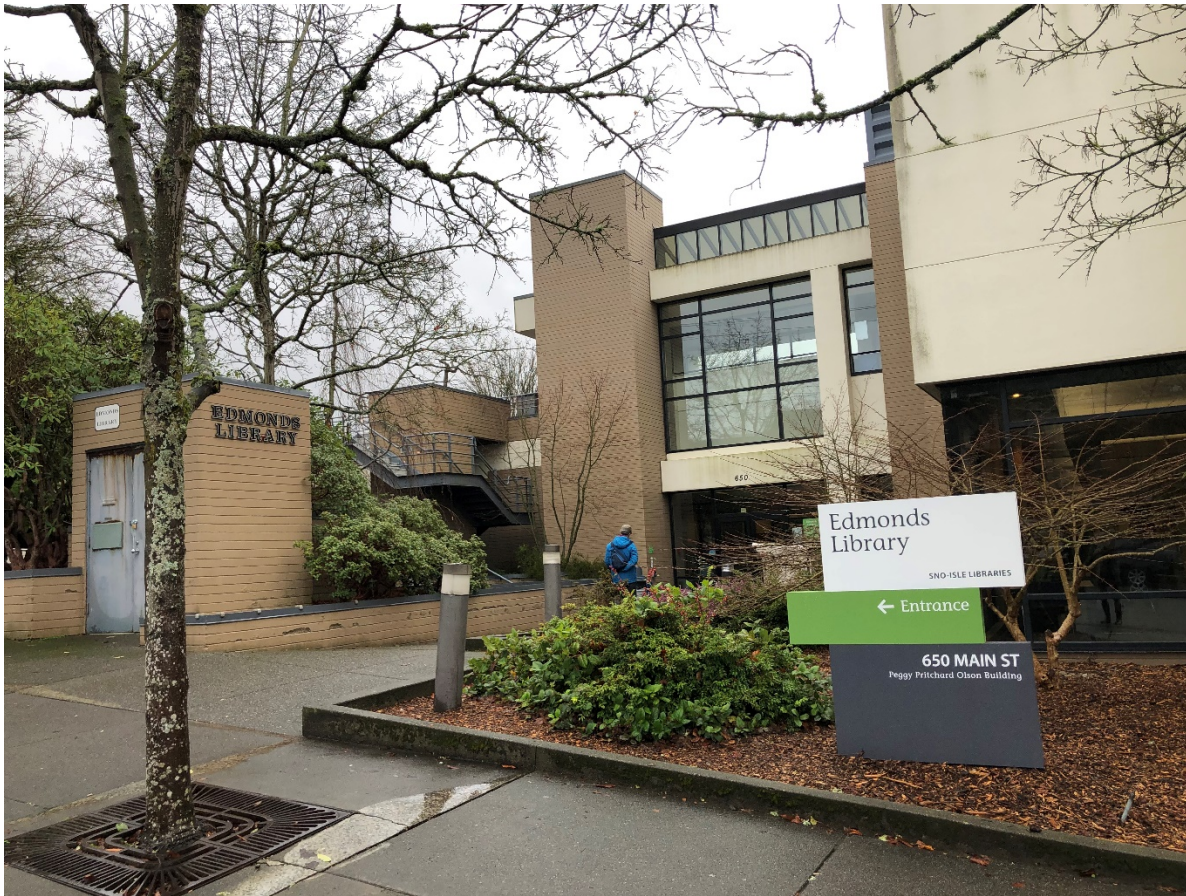
Front view of existing site at 650 Main St.
